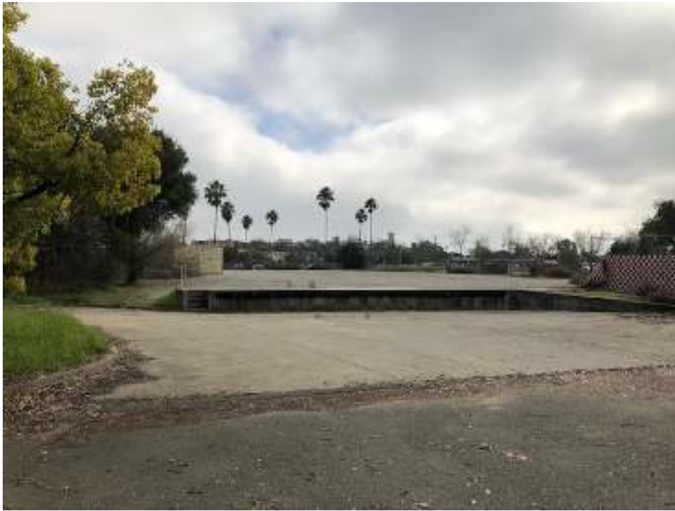
Figure 10: Looking east across the site towards C Street (existing loading dock onsite in foreground)
