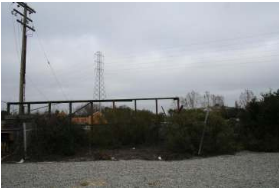
Figures 6 and 7: Views from the Project Site to the north towards apartments under construction across State Access Road
