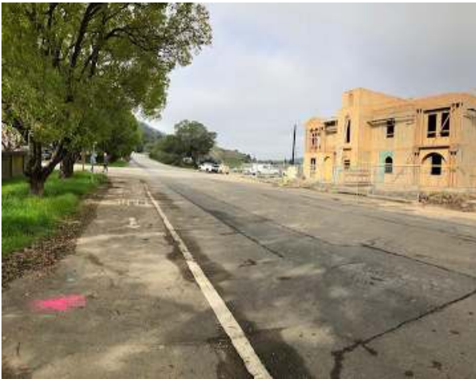
Figure 13: View looking west down State Access Road (Project Site is south and apartments under construction are north of the road)
