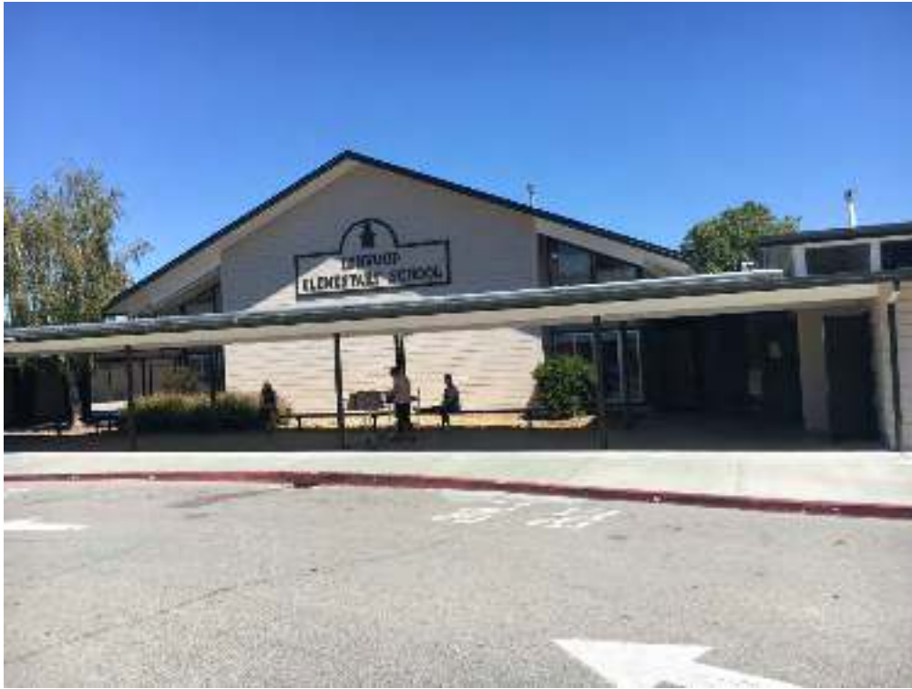
Figure 7: View of Lynwood School from Existing Entry Area
